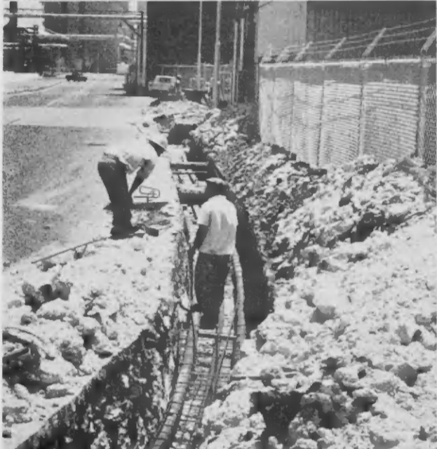
WORKMEN LAY reinforcing steel in a ditch near No. 1 Powerhouse for transformer cable conduits, then fill the ditch with cement. Top photos show general views of the transformer installation.
